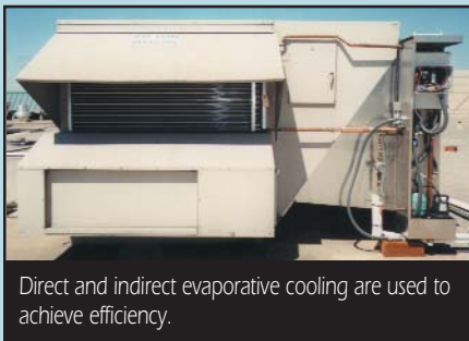
Dual Cool system provides roof top air conditioning units with a boost in capacity and efficiency.
