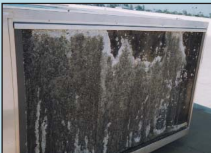
Clogged media caused by poor water quality in test areas leads to increased maintenance issues.
