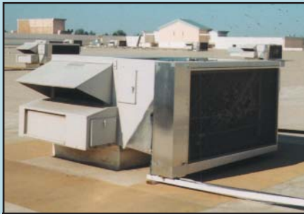
Dual Cool system provides roof top air conditioning units with a boost in capacity and efficiency.
