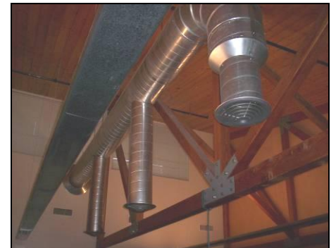
Figure 10: The project team decided to install new ductwork for the Coolerado. Photo credit: ADM Associates Inc.
