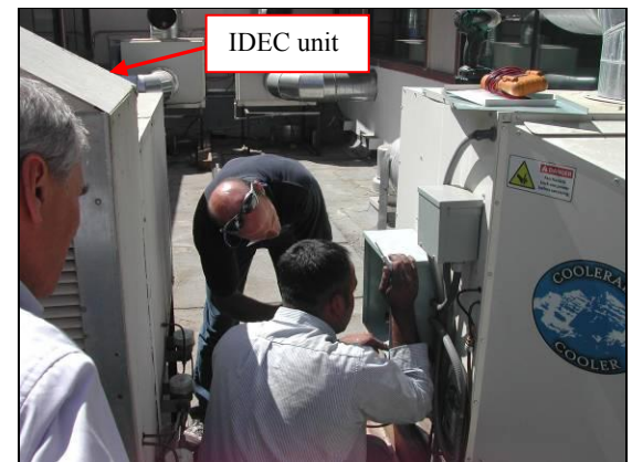
Figure 7: Crew installing the controls for the new unit. Note the IDEC immediately next to the Coolerado.
