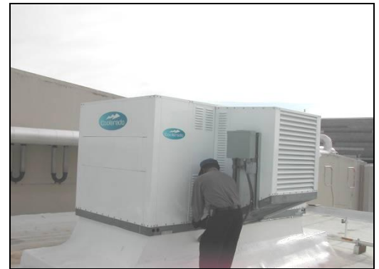
Figure 27: Coolerado's H80 Hybrid Air Conditioner.
