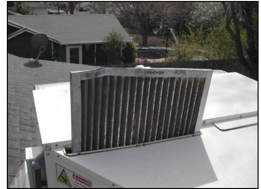
Figure 21: If the Coolerado is installed on a rooftop, it may be easy to forget to change the air filters on a regular basis.
