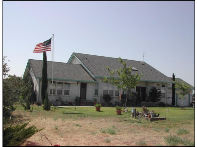
Figure 5: In retrospect, expecting one Coolerado R600 to provide adequate cooling for an older 2,600 square foot home with two stories and no exterior shading in Sacramento was overly optimistic.
