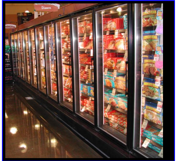
Figure 6: Freezer cases illuminated with Hussmann Corporation's new LED lighting system.
