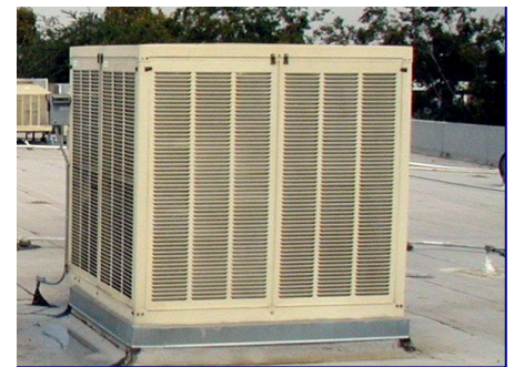
Figure 2: Fiber-pad direct evaporative cooler with aspen pads
