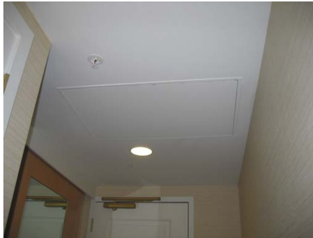
Figure 4: Hotel #1 Fan-Coil Unit Ceiling Access Door
