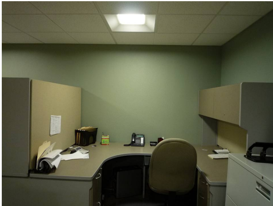
Figure 1: CREE LR24 LED Troffer In Open Work Space
