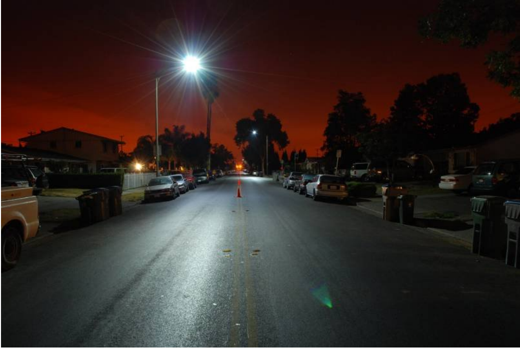
Figure 23: Street Level Shot, LED 75%
