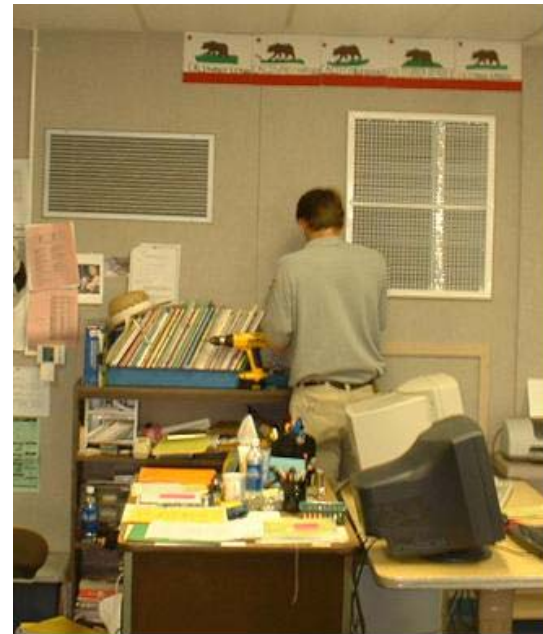
Left photo: OASys mounted on outside wall, adjacent to conventional HVAC unit. Right photo: supply register on inside wall
