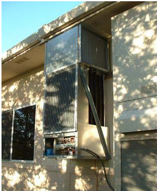
Left photo: OASys mounted on outside wall, adjacent to conventional HVAC unit. Right photo: supply register on inside wall
