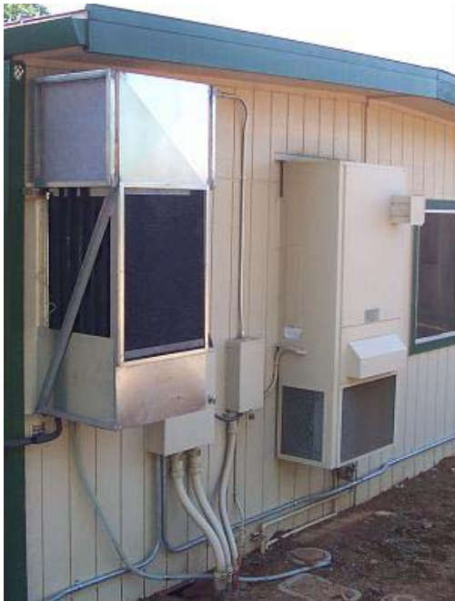
Left photo: OASys mounted on outside wall, adjacent to conventional HVAC unit. Right photo: supply register on inside wall (tears in tackboard are pre-existing).
