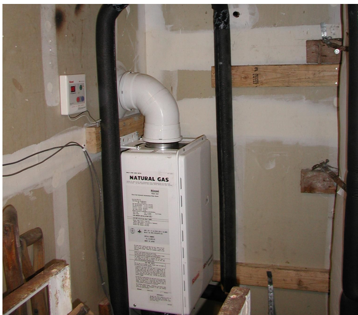
Figure 1: Garage Sidewall Tankless Installation
