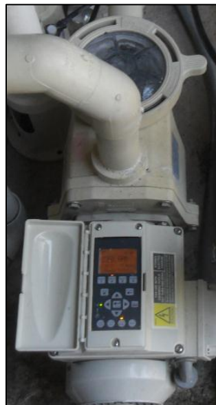
Figure 1: Variable Flow High Performance Pool Filtration Pump
