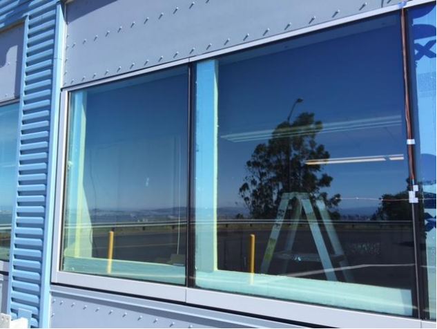
Paneling for lower window-to-wall ratio
