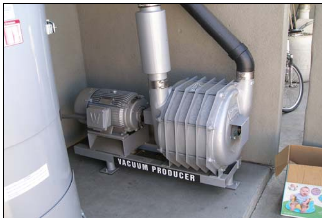
FIGURE 1. CENTRIFUGAL VACUUM PRODUCER
