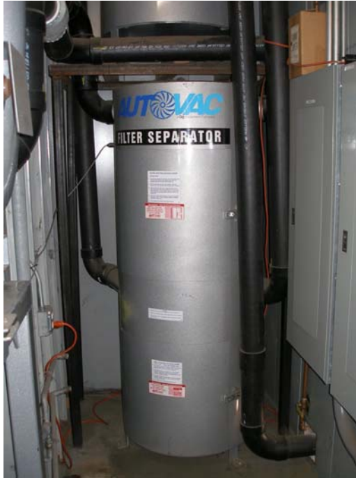
FIGURE 3. FILTER SEPARATOR
