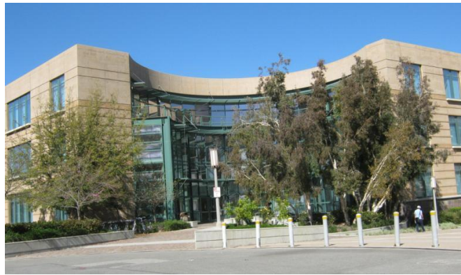
FIGURE 15. NATURAL SCIENCES I BUILDING
