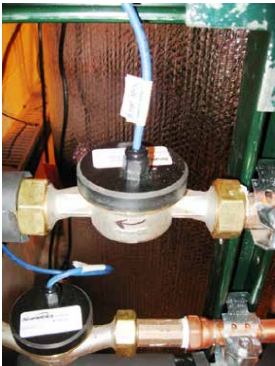
Figure 6 300 Pulses per Gallon Water Meter
