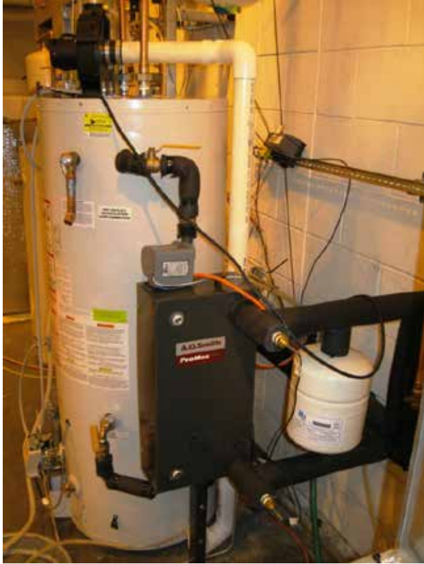
Figure 4 High Efficiency Water Heater with Side-Mounted Heat Exchanger for Panel Hot Water Supply
