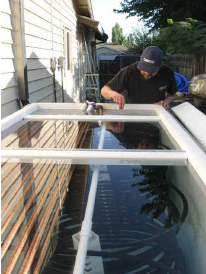
Figure 15 Chilled water storage tank in Grandstaff house
