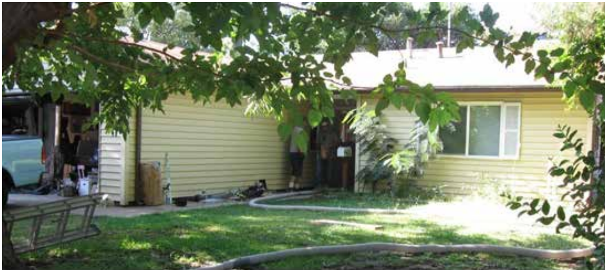
Figure 2 Grandstaff field test house
