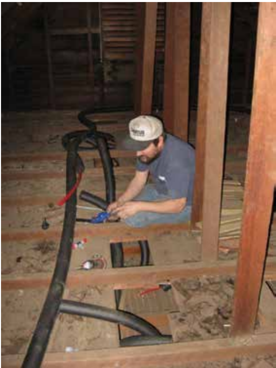
Figure 18 Tubing installation in the attic of the 6th Avenue house
