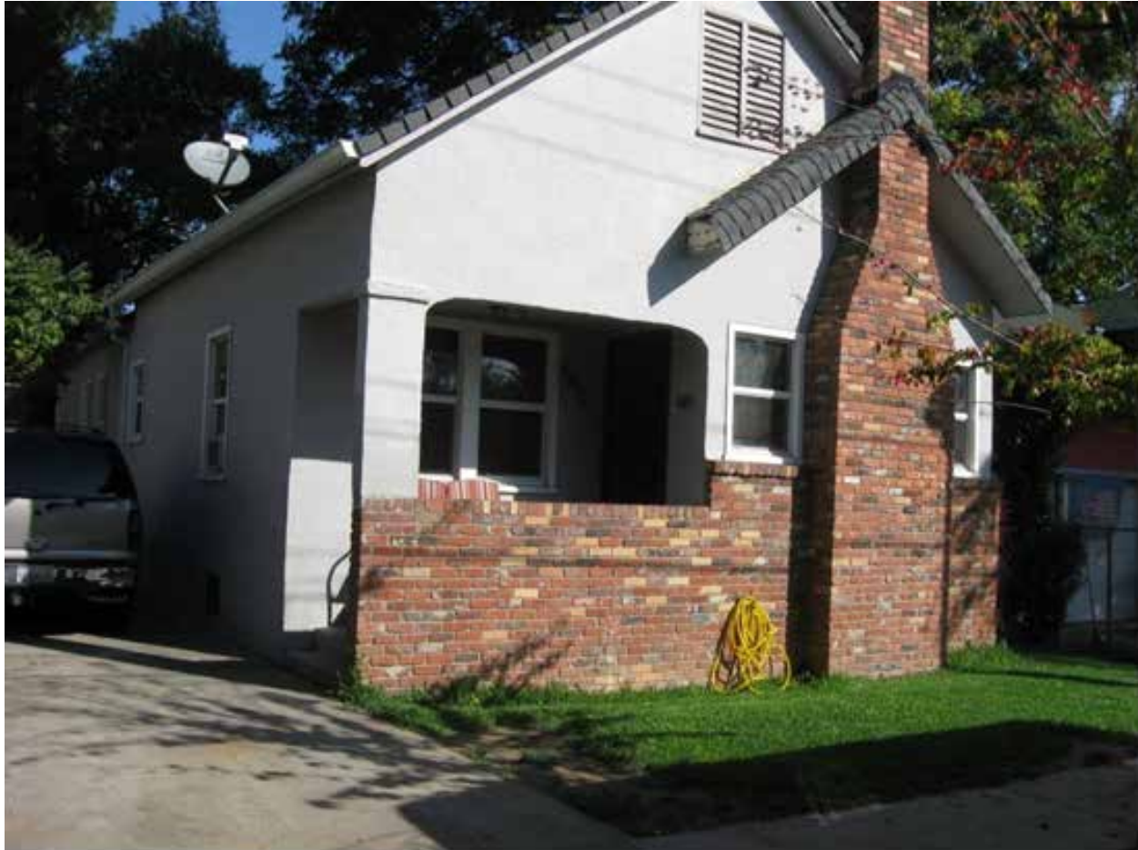
Figure 4 6th Avenue Field Test House
