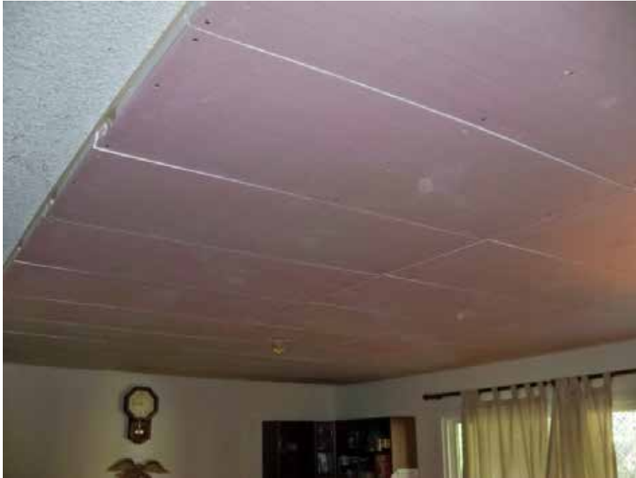
Figure 12 Uponor panels installed in the Grandstaff house
