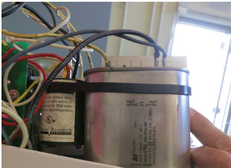
FIGURE 6: MULTI-TAP CAPACITOR – BASELINE MH AS FOUND: INCORRECTLY WIRED FOR 15 \mu\text{F}
