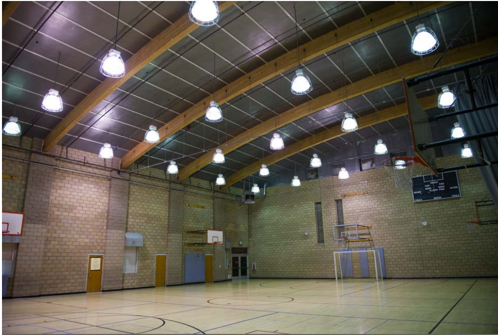
FIGURE 1: BASELINE MH LIGHTING IN THE GYMNASIUM - PHOTO TAKEN AT 4000K EXPOSURE SETTING
