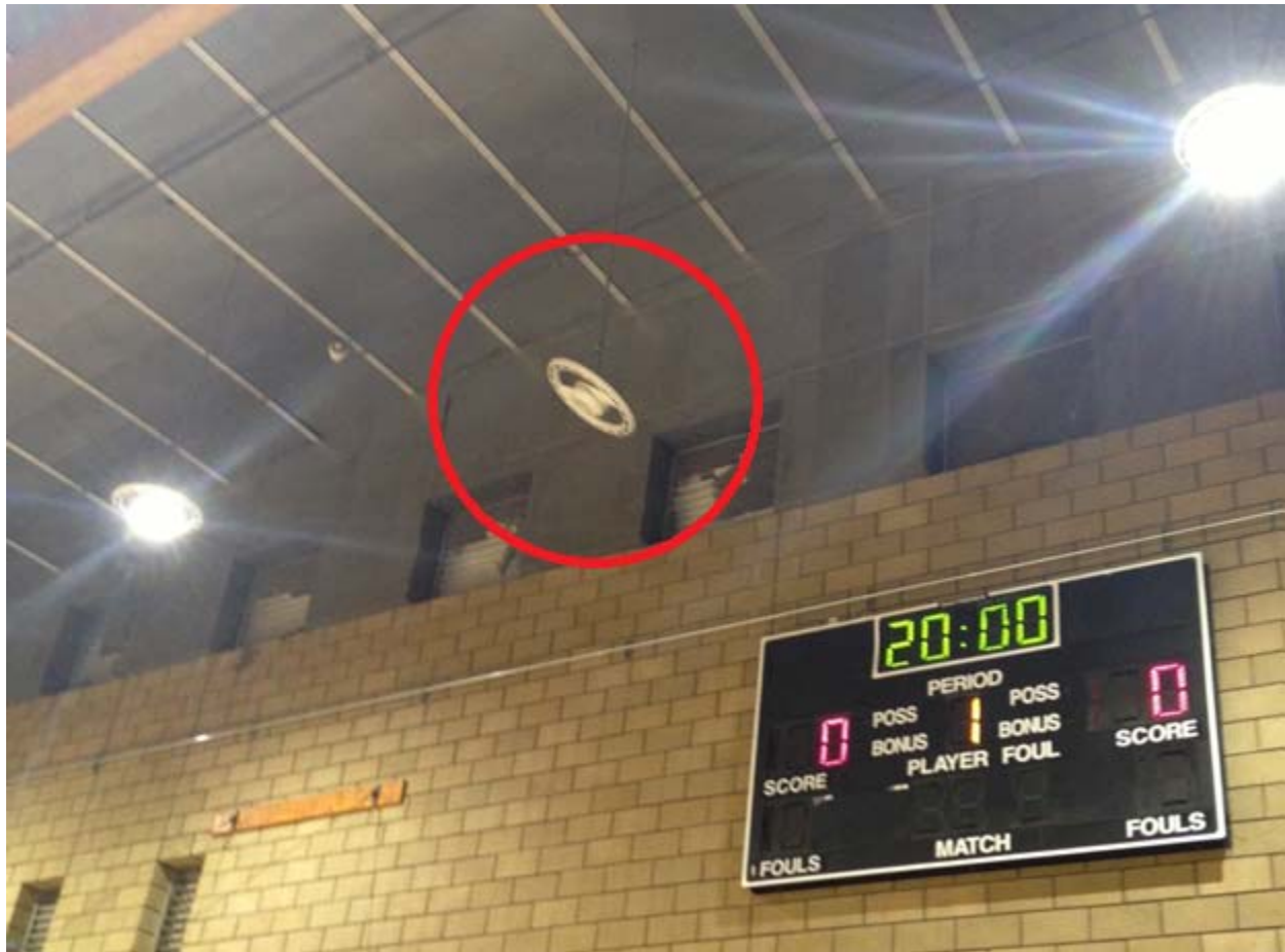
FIGURE 11: FAILED LED FIXTURE
