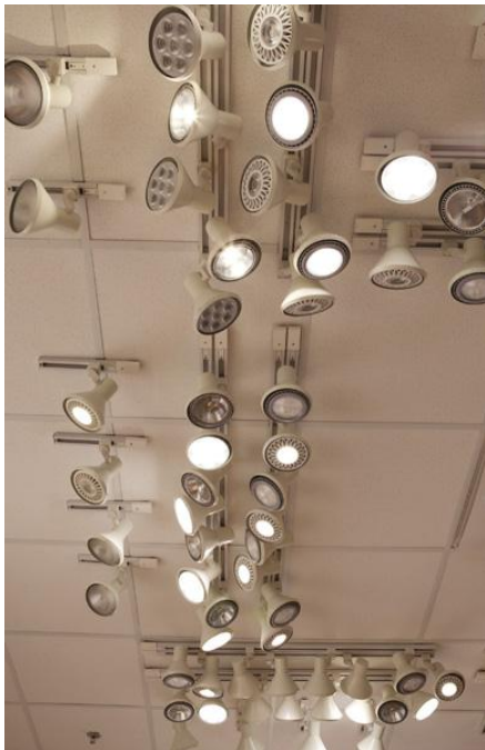
FIGURE 6. LED PAR 38 LAMPS IN TRACKS IN LUX
