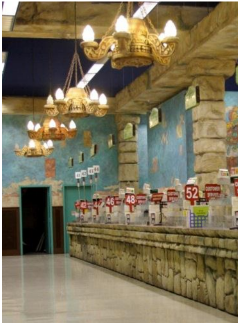
FIGURE 7. 60W INCANDESCENT A LAMPS WITH STANDARD SCREW BASE IN SUSPENDED CANDELABRA CHANDELIER
