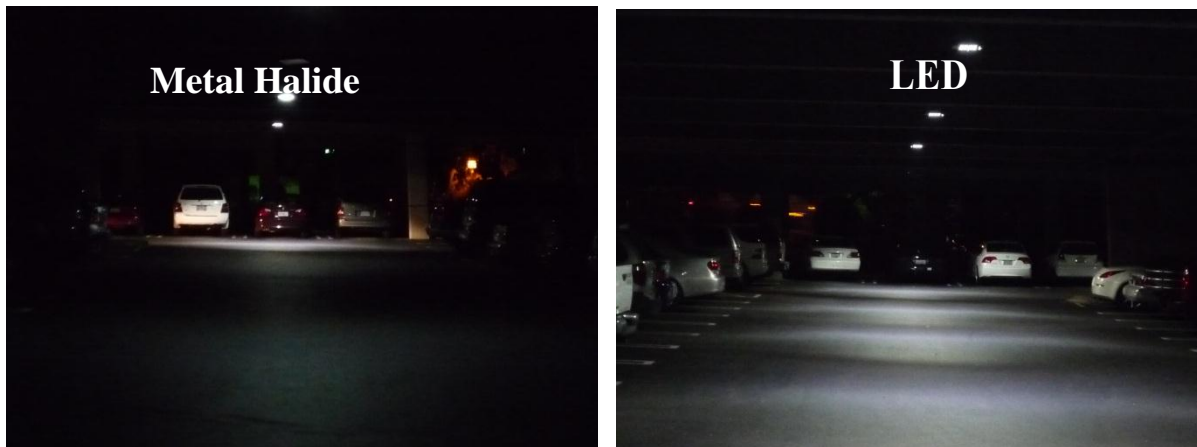
Figure 3: Metal Halide lane (left) vs. LED lane (right)
