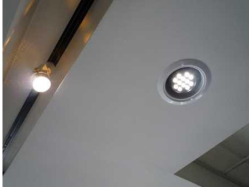
Figure 4: Unobtrusive light – recessed into the ceiling
