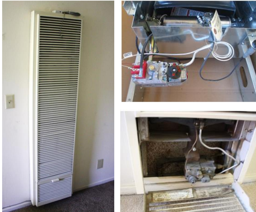
Figure 3 - Typical wall furnace, new control valve, old control valve
