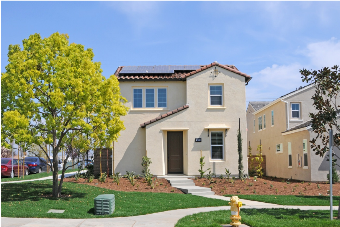
FIGURE 6. CONSTRUCTED ZNE NEW HOME
