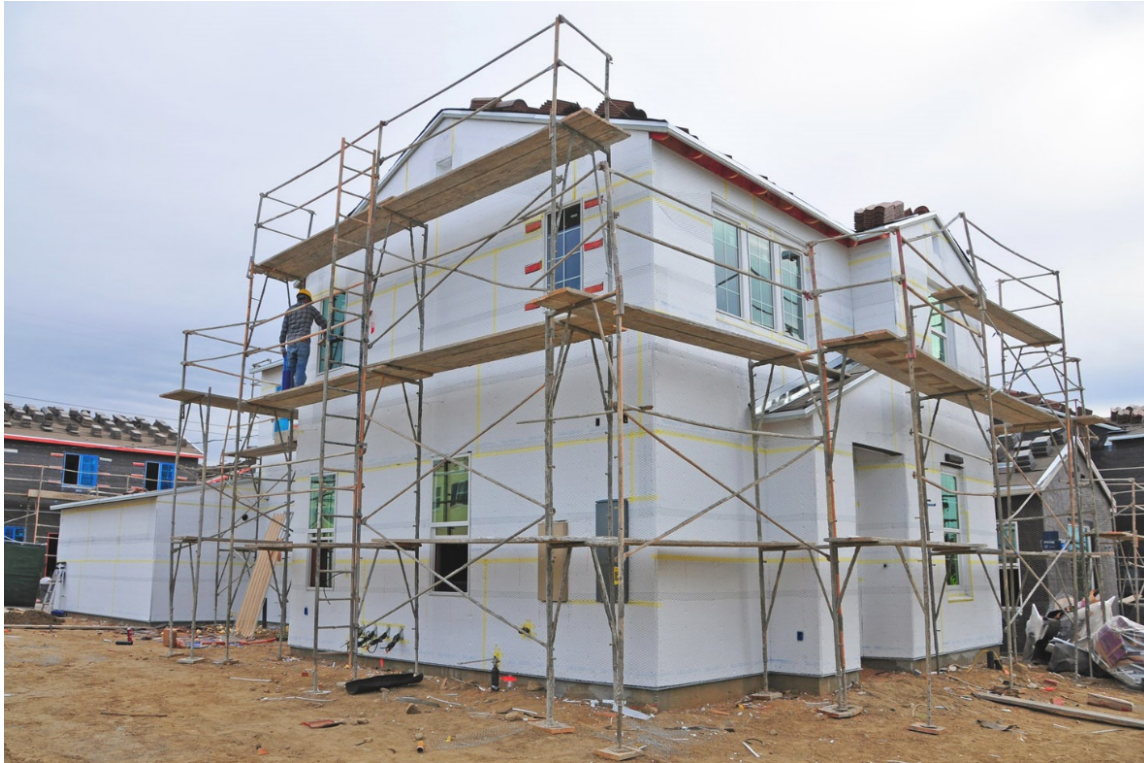
FIGURE 5. ZNE HOME DURING CONSTRUCTION
