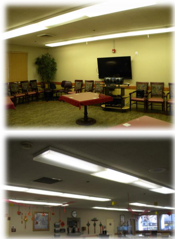
Figure 5: Although the original lighting system was fairly energy efficient, it was very industrial looking and could not be dimmed. This did not provide many options for controlling the lighting during the various activities taking place in the dining room.
