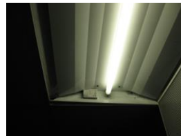
Figure 5: The original lighting system had been de-lamped as part of a previous energy efficiency project
