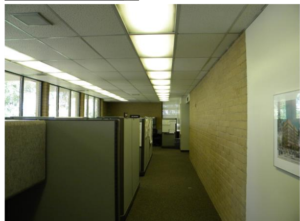
Figure 5: The original lighting system had been de-lamped as part of a previous energy efficiency project
