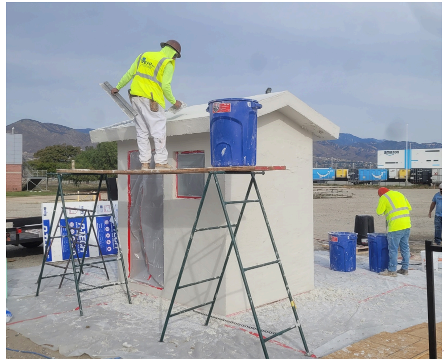
U-Stucco being installed.
