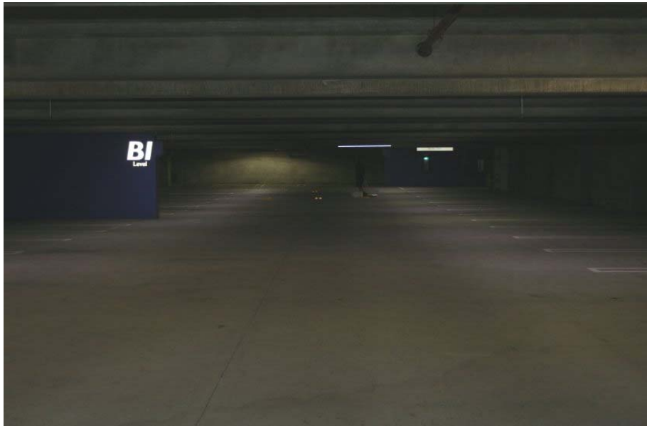
FIGURE 3: POST-INSTALLATION COLOR TEMPERATURE
