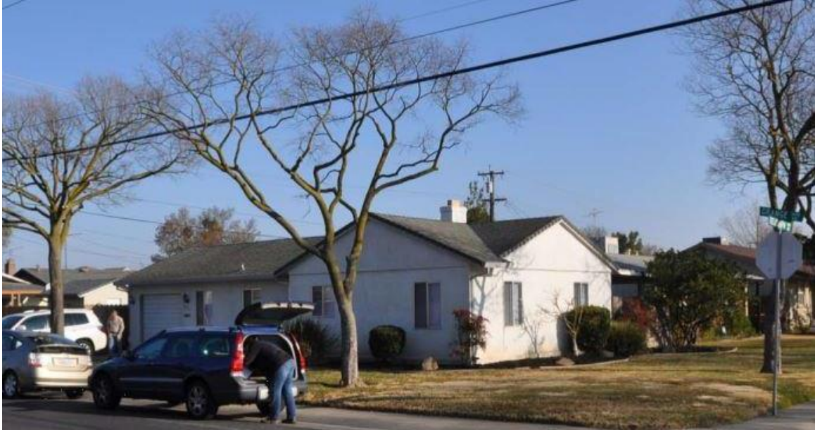
FIGURE 7. GRANGE TEST HOUSE
