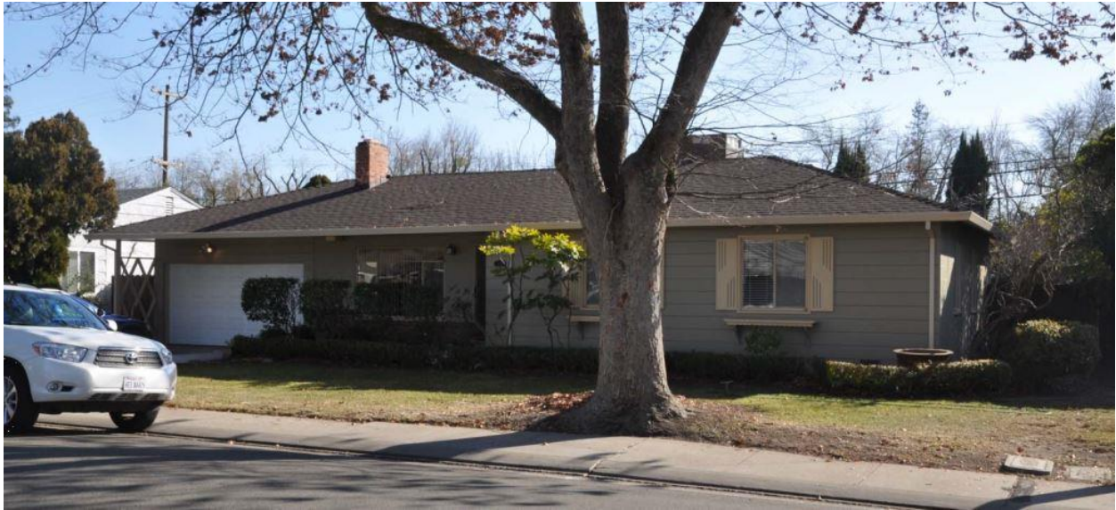
FIGURE 8. MAYFAIR TEST HOUSE - FRONT
