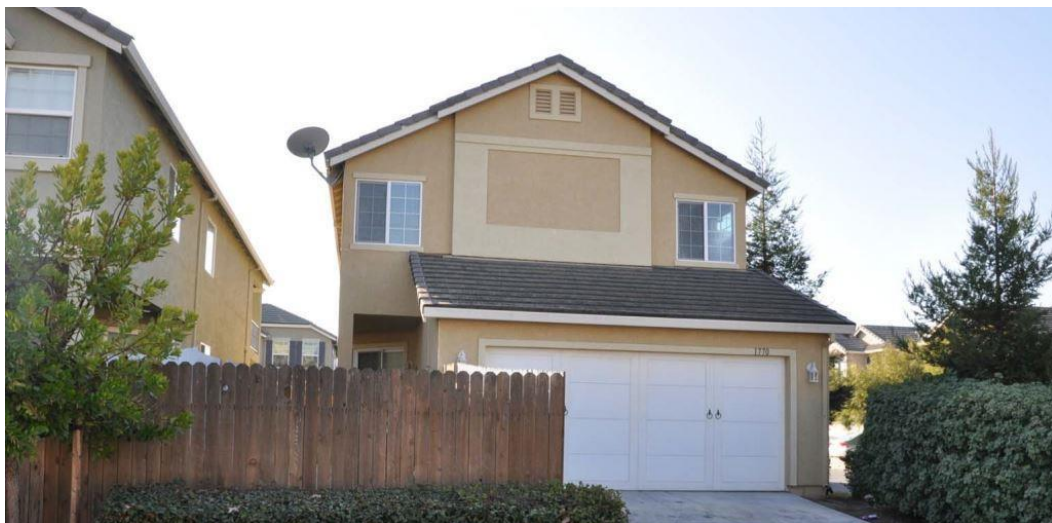
FIGURE 6. CALEB TEST HOUSE – REAR VIEW
