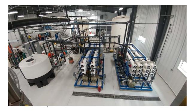
Dewatering of solids and replacement with RO Reject provides high strength fuel to an Anaerobic Digesters
