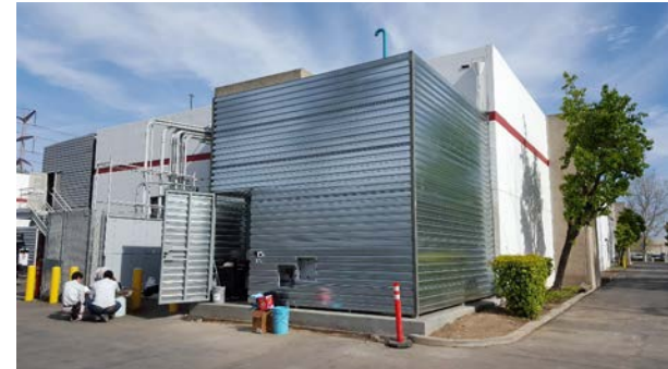
New outdoor mechanical area
